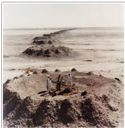
Figure 15: Qanat lines of boreholes and weirs to evenly distribute brine without eroding the flat desert
