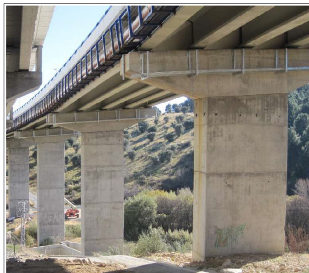
Figure 7: Metal Walkways installation for the Viaduct Maintenance [12].
