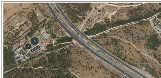
Figure 2: Aerial Photograph of La Jarosa Viaduct (Photograph from the Spanish National Geographic Institute)
