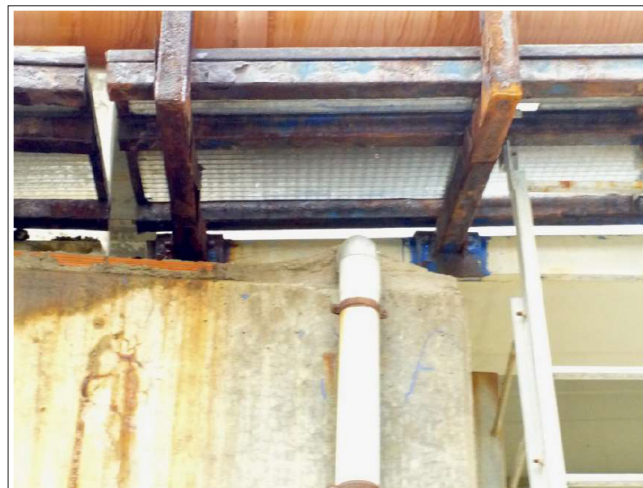
Figure 13: Detail of the Area Photographed in Figure 12, Where the Corrosive Phenomena Can be Observed in Greater Detail (Photograph Taken with the Anafi Parrot Drone)
