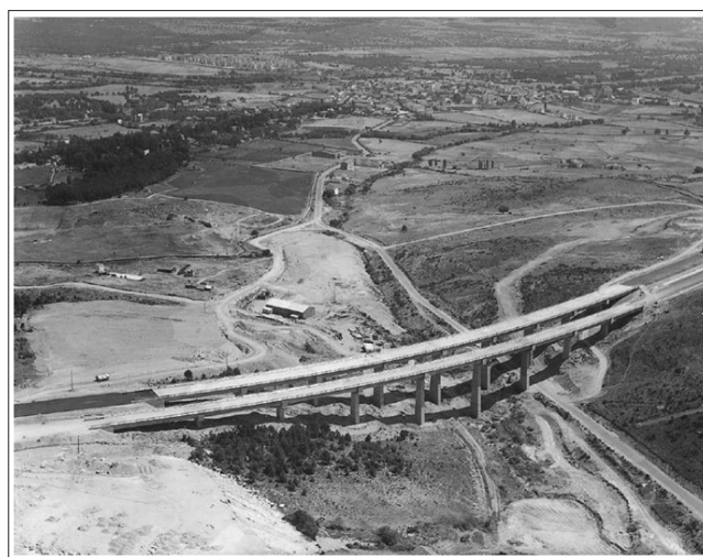
Figure 3: Aerial photograph of the La Jarosa Viaduct image taken at the second structure conclusion (photography by Juan José Jover) [10].
