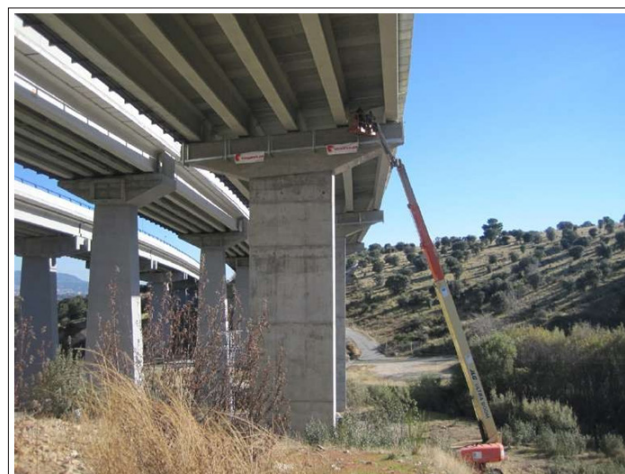
Figure 6: Metal Walkways installation for the Viaduct Maintenance [12].
