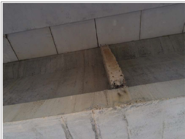
Figure 10: General View of a Concrete Brace, Arranged in the Web of a Precast Beam (Photograph Taken with the Anafi Parrot Drone).
