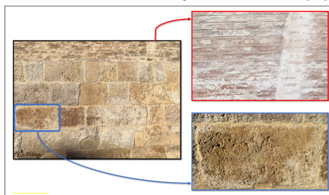
Figure 8: Detailed Optical Analysis of the Two Materials that make up the Masonry of the Giralda Bell Tower: Calcarenite at the Base and Ceramic Brick with Mortar (Photographs by the Author on Different Points of the East Facade)
