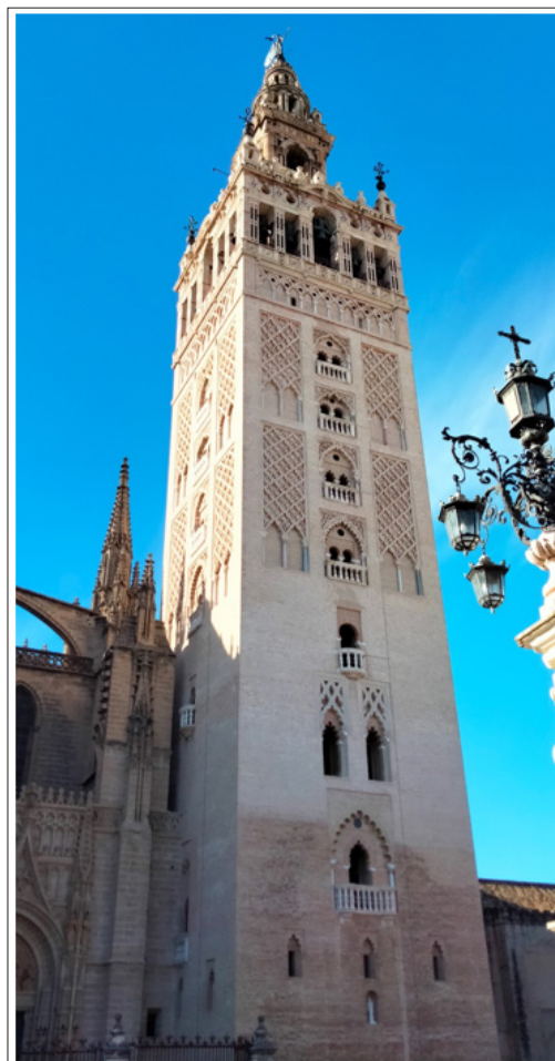
Figure 1: East facade of the bell tower Giralda (photograph by the author)
