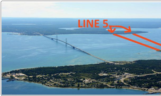
Exhibit 8: Line 5 pipeline system underneath the water (URL6, 2020, : https://images.app.goo.gl/NeXiMe3MuxWlRvpx9 )
