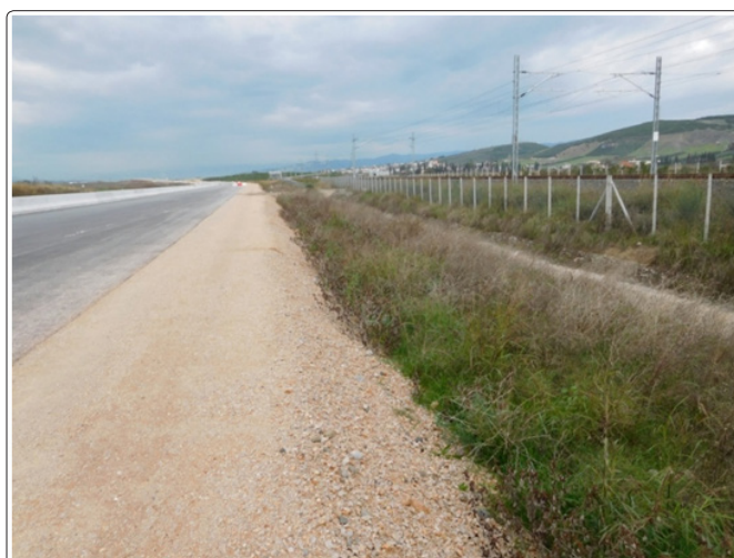
Figure 3: Stretch of Motorway E65 in Central Greece: low risk of wildfire
