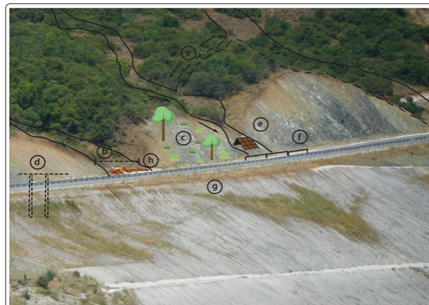
Figure 4: Preventive and protective measures against road inundation: preventive (a) watercourse diversion, (b) watercourse widening (c) additional vegetation uphill (d) intercepting pits and wells, protective (e) intercepting steel racks upstream (f) removable waterproof panels (g) slopes reinforced by geotextiles (h) removal of debris from culvert inlet.
