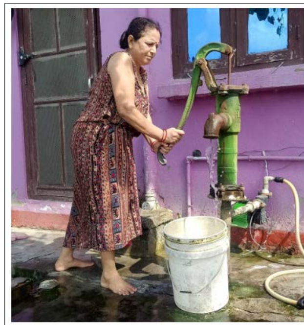
Figure 3: Suction Hand Pump for Domestic Purposes
